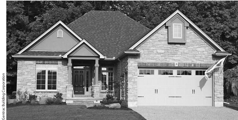
Figure 4.2. The 1,530 square foot Merlot model green home, built by Gentrac Building Corporation, consists of a 785-watt Sanyo solar array. The system also has a backup power system, which can, during power interruption, supply designated essential circuits about three days worth of electricity.
